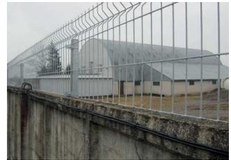
**Light welded mesh fence (Fig. 8)**
